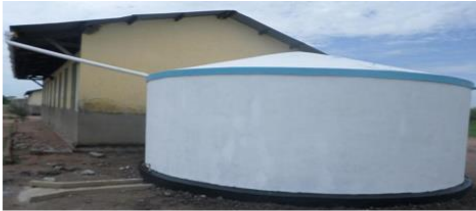
Figure 3. Rain water harvesting tank constructed
