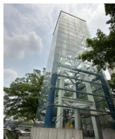
Figure 5. Amber Water Tower.
