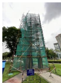
Figure 6. Skeleton Water Tower Current Status.
