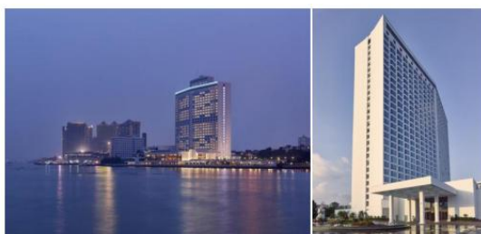
Figure 1. White Swan Hotel exterior view. Source: https://image.baidu.com
