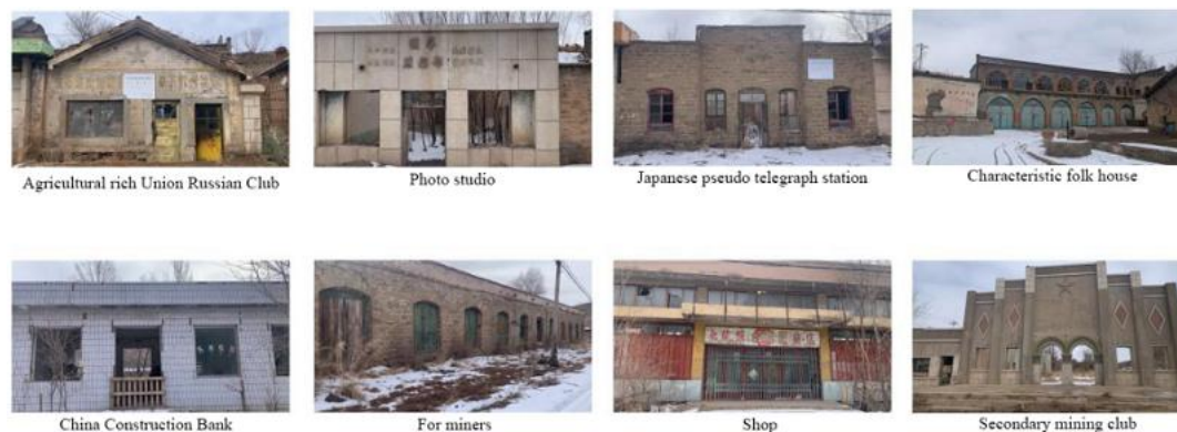
Figure 1. Current status of architectural remains in Dafa Old Street.
