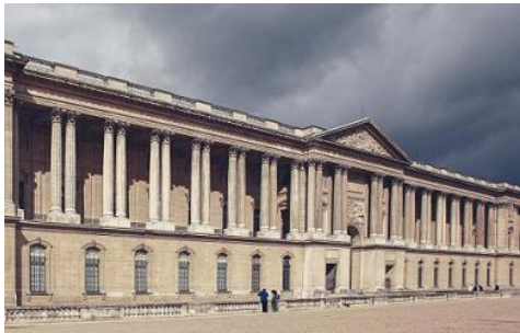
Figure 17. East Façade of Louvre Official Building.
