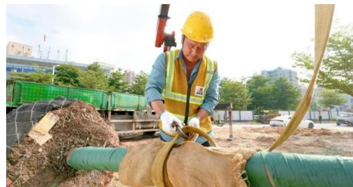
Figure 10. Lashing before hoisting.
