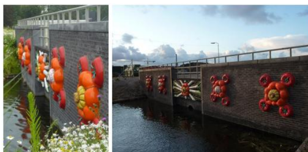
Figure 5. Ceramic relief on the culvert.
