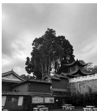
Figure 2. Caoxi Temple Architectural Complex.
