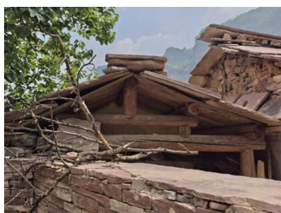
Figure 5. Post-and-lintel Wooden Roof Truss.
