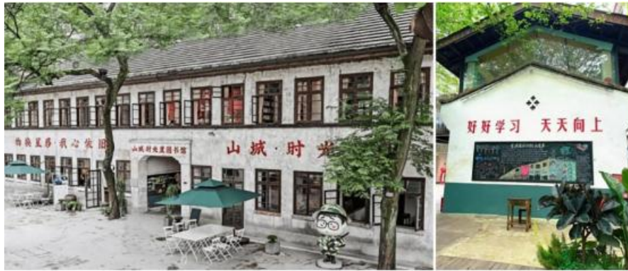
Figure 3. Renovation of Jinmasi Primary School in Shancheng Lane.
