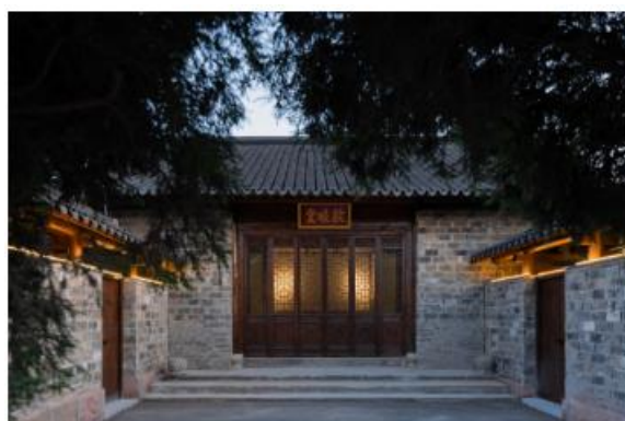
Figure 2. Fan Clan Ancestral Hall renovation and renovation.
